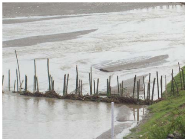
Constructing bamboo porcupines is common as a flood protection measure in Dhemaji on river Subansiri
