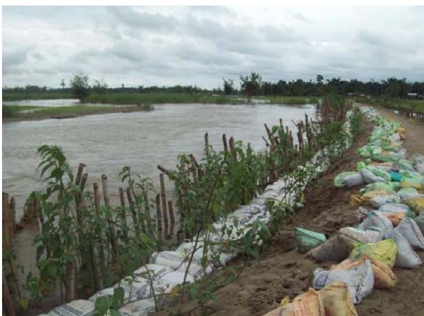
Channels shift so abruptly in Dhemaji that the entire district can be considered a flood plain of a river. Bunds are being used as a flood protection measure here through support of RVC and NREGA programmes.
