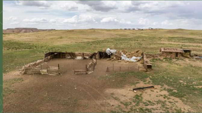
Photo 1: Herder P's winter shelter collapsed due to the explosions made by the eight mining companies nearby, making it impossible to bring livestock inside. Photo: P (anonymous)
